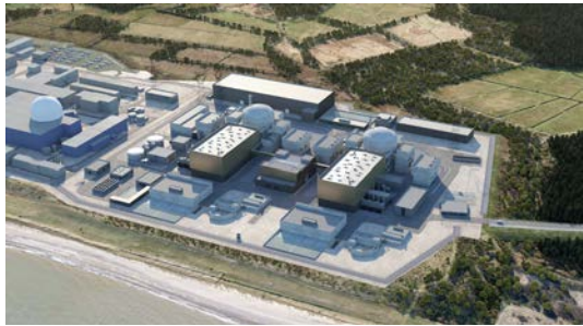
Aerial view of Sizewell C Operational Site
