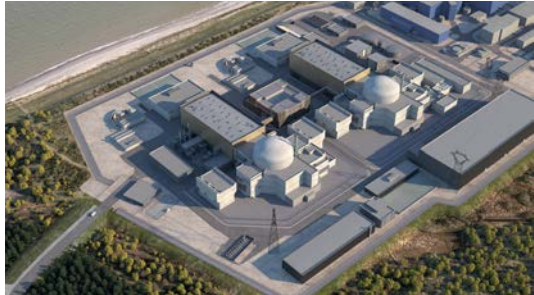
UK EPR™ Safety related buildings aerial view
